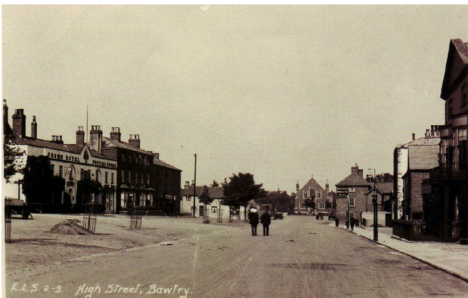
When almost all roads were unsealed: Bawtry around 100 years ago.
